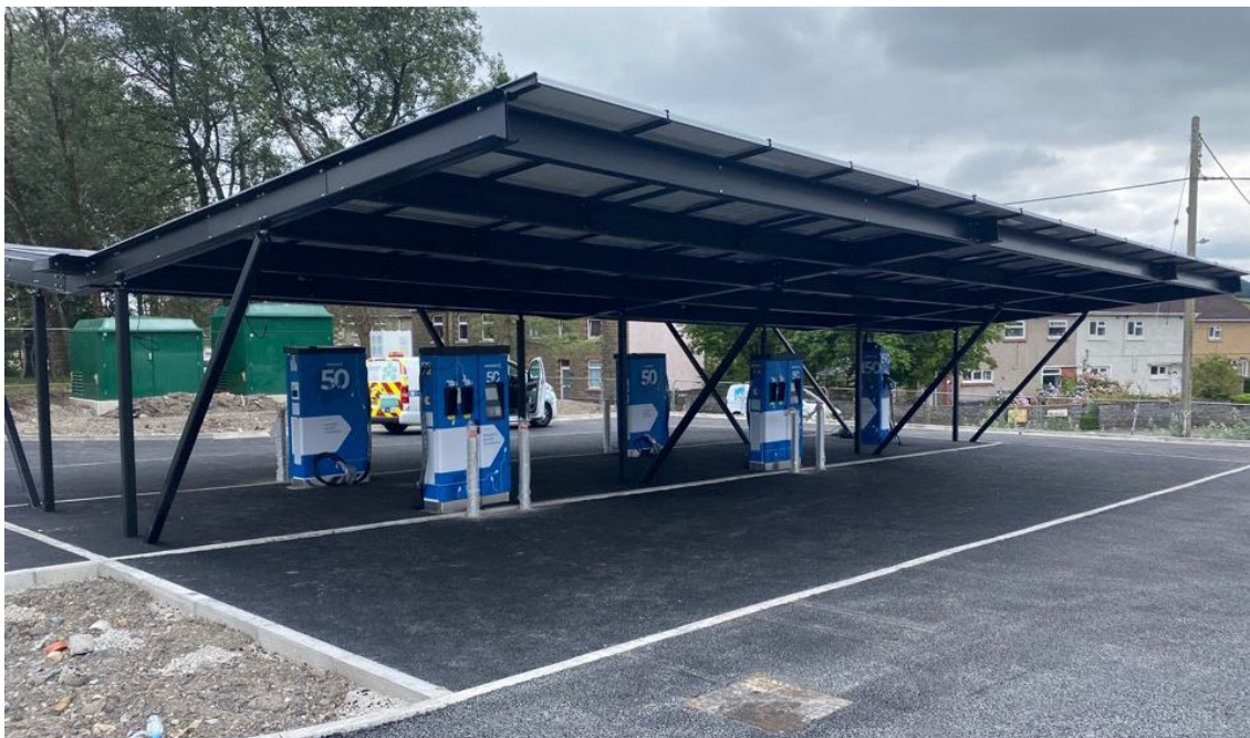
Figure 16 - Cross Hands EV Charging Hub (in construction)
